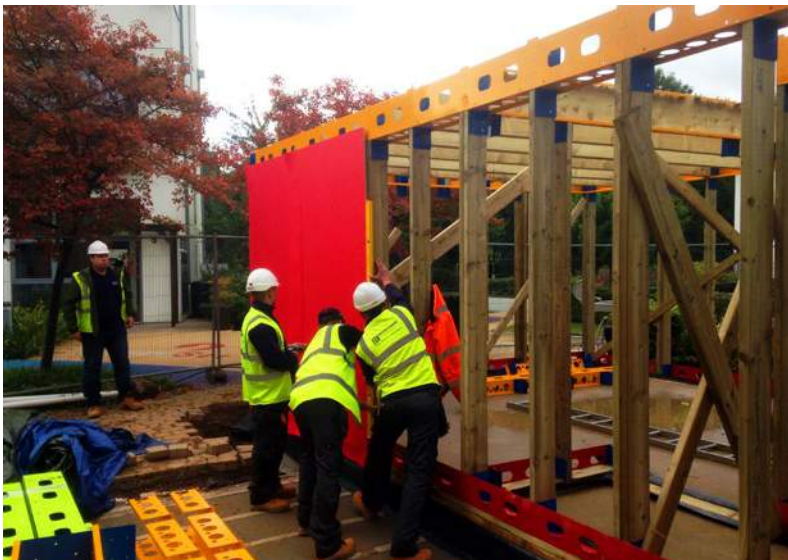
Self-adhesive airtightness and weather proof membrane bonded to OSB board and then fixed to timber studs
