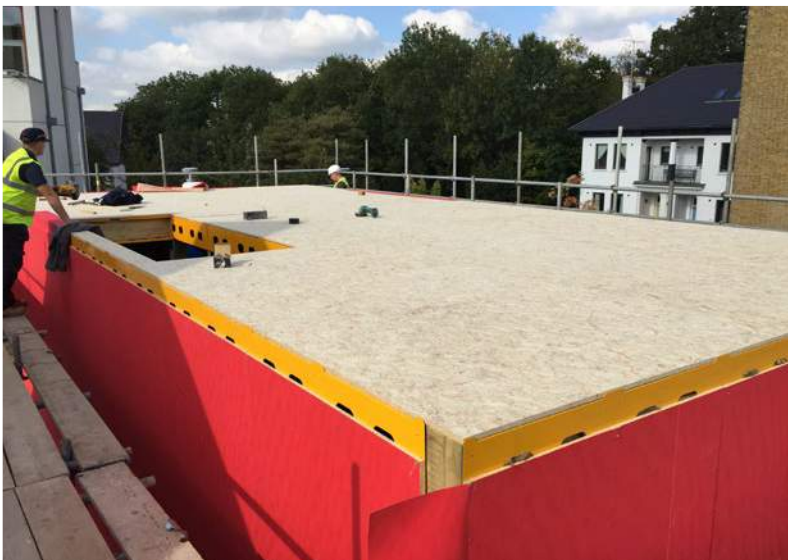
OSB fixed to floor joists
