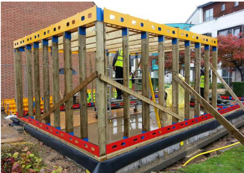
Factory cut steel easily combined with timber studs sourced through local builders merchants
