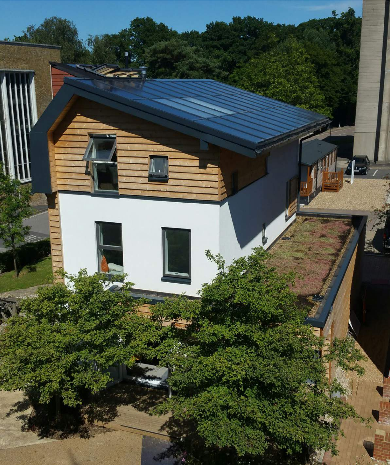
▲ 7.5kW peak HiminZED BIPV roof at BRE Innovation Park
