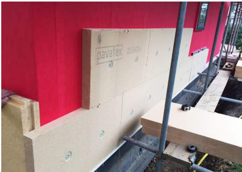
Breathable external insulation skin removes thermal bridges
