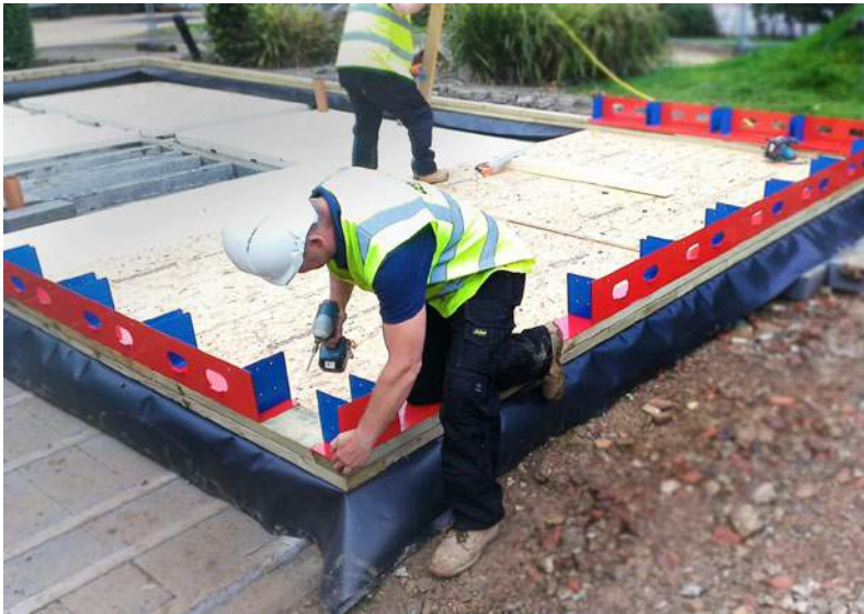
Factory laser cut steel structural ring beam
