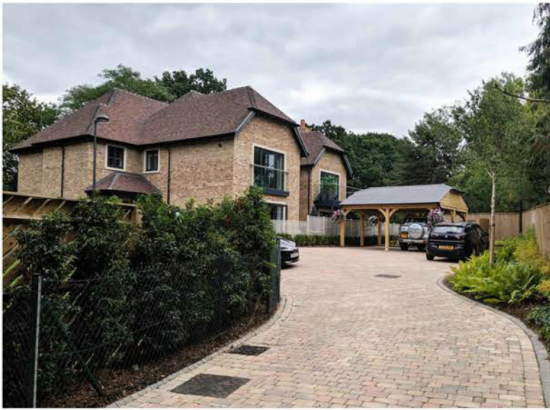
Views of front of car port
