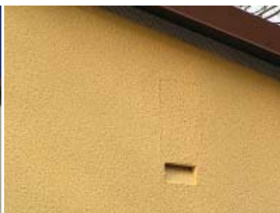
Schwegler 1FR Bat Tube, to be integrated into building wall, and either bricked in or rendered. Self-cleaning. Dimensions: 47.5 x 20 x 12cm.
