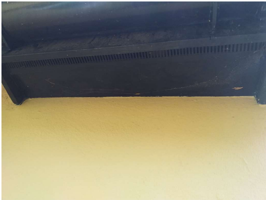
Tight seal on house soffit
