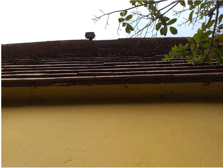
Seal between render wall sections and tiles.
