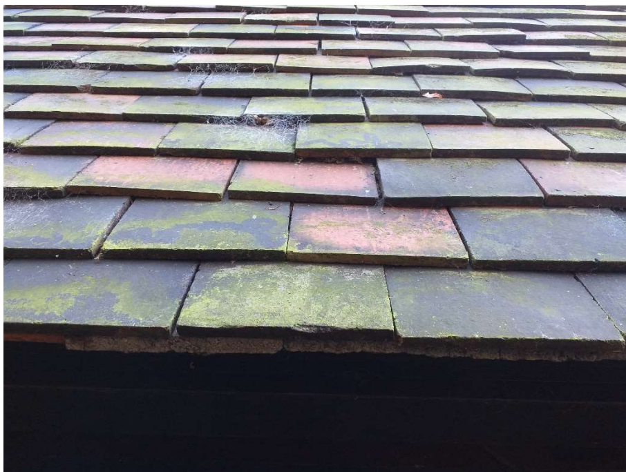
Indicative section of hanging tiles. Note absence of lift and cobwebs
