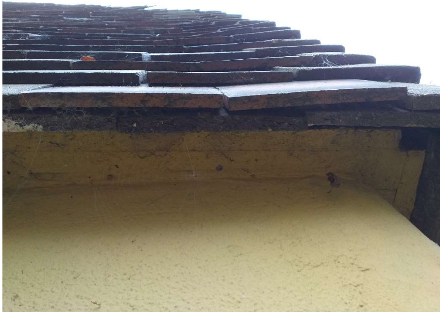
Indicative section of hanging tiles. Note absence of lift and cobwebs
